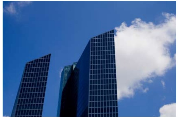
Munich Business Towers
