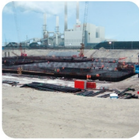
Reinforcement works for Power Island raft foundation
